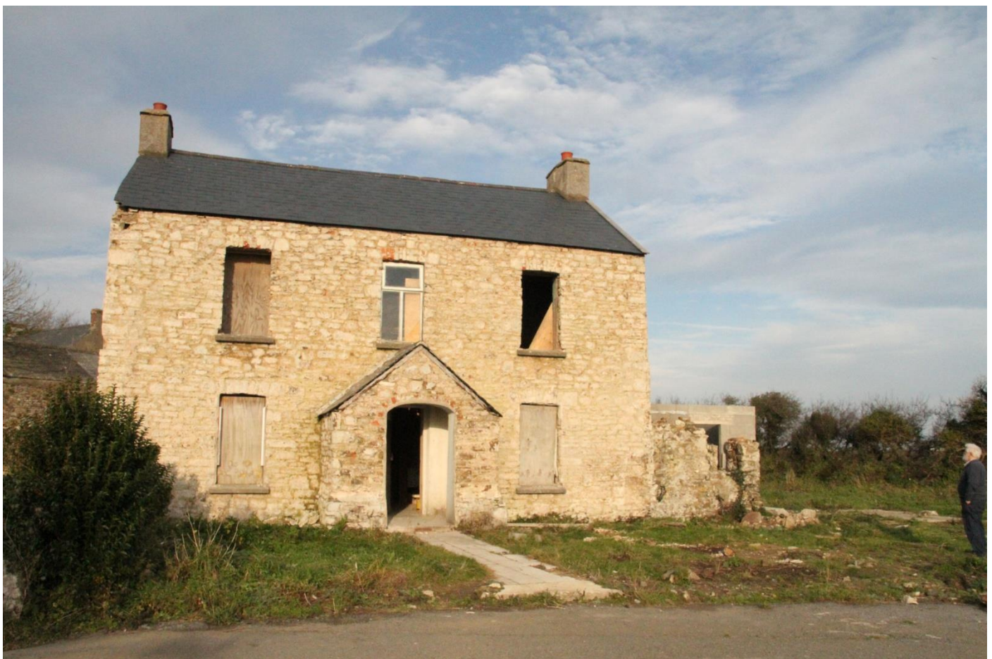
Ready to start the next phase (December 2014)
