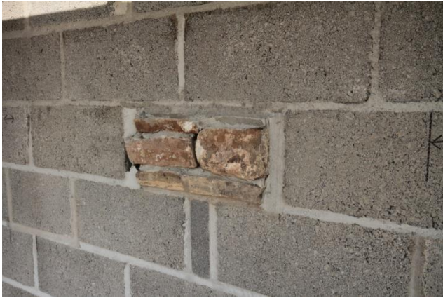
The extension have breeze block walls while the interior is lined with softwood frames
