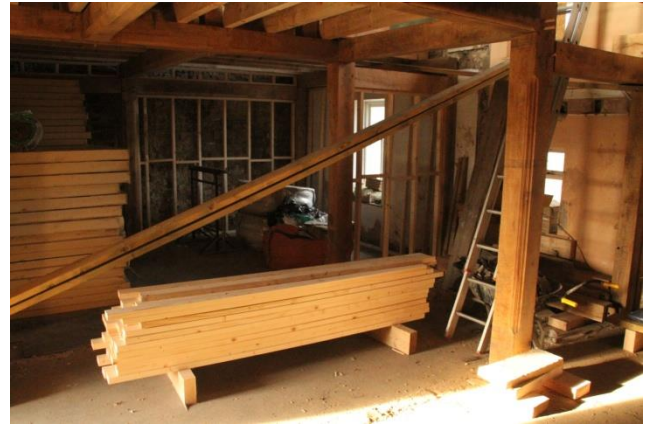
The extension have breeze block walls while the interior is lined with softwood frames
