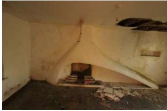
The chimney place turned out to be all that was supporting the first floor
