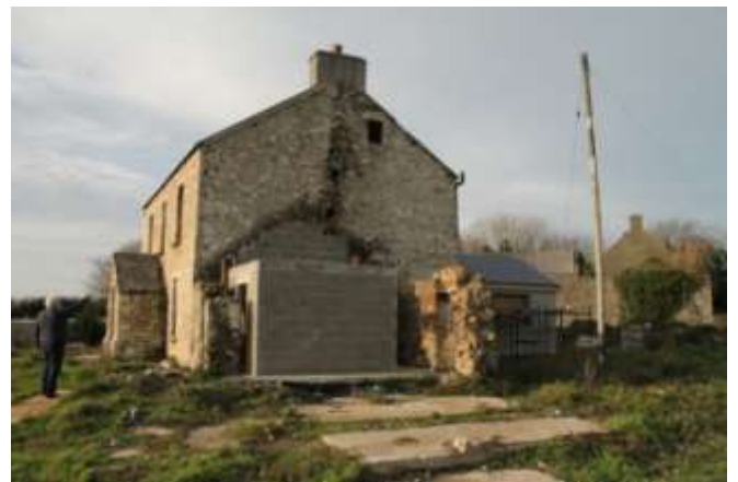
The interior was gutted and the chimney supported with buttresses (now the downstairs bathroom)
