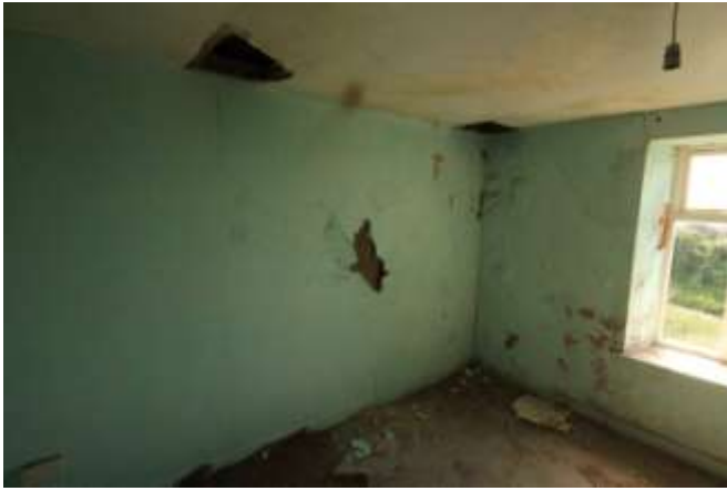
The chimney place turned out to be all that was supporting the first floor
