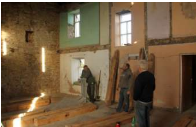
The interior was gutted and the chimney supported with buttresses (now the downstairs bathroom)
